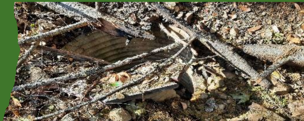
Plugged Culvert
